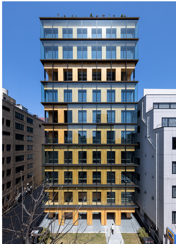
FIGURE 3: PortPlus is Japan's first fully wooden and fire-resistant high-rise structure: it is a 10-story building in Yokohama completed in 2022, designed and built by zenecon Obayashi ( https://www.oyproject.com/photos/ . Photographer: SS Inc.).
